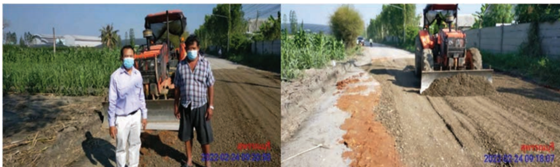
Photo : Bring gravel and stones to repair and improve Wang Nam Joan road.
